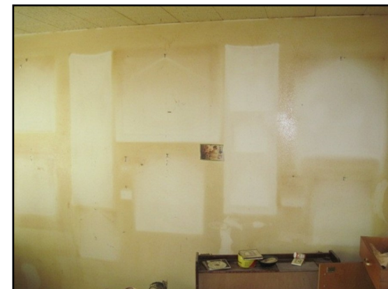
A home where family members smoked inside. This shows the wall once pictures were removed. Nicotine and smoke chemicals stay on the wall.
